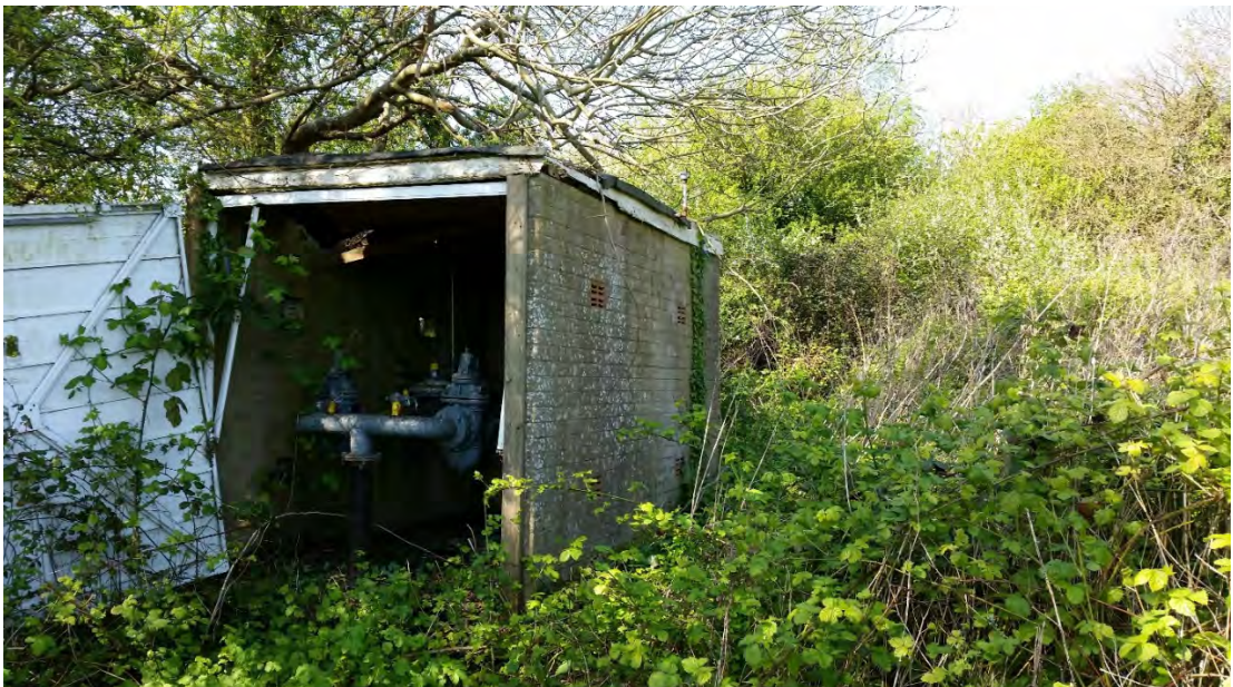
Photo EDP 10: Derelict building located within south west corner of Field I surrounded by dense scrub.
