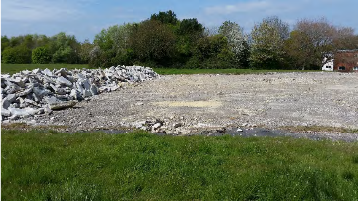
Photo EDP 11: Demolished remains of former school.
