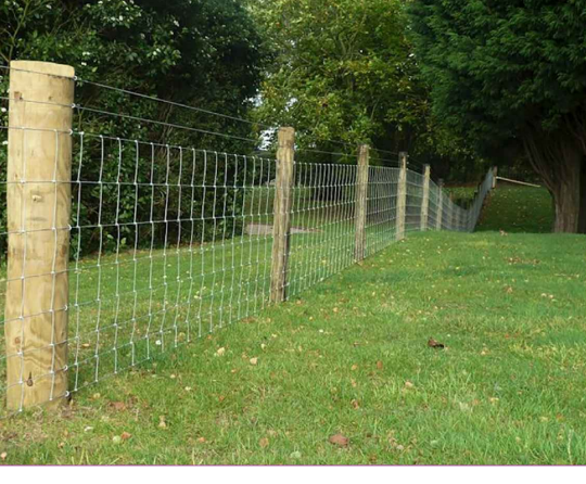
Protective Fencing for Dormouse Habitat
