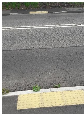
Plate 3.2: Dropped kerb and tactile paving crossing facility
