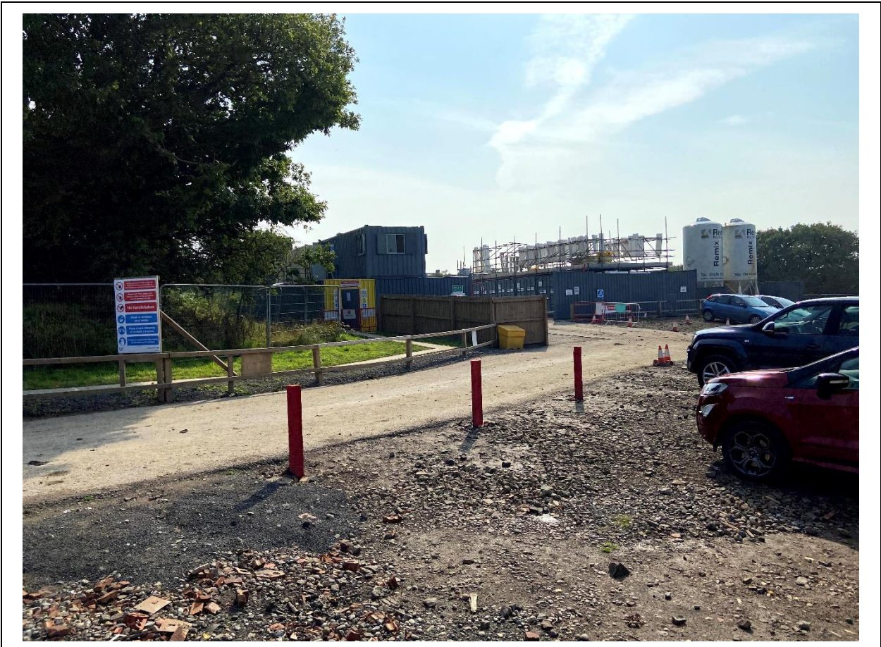
Plate 1: View south-east of the entrance to the Site.
