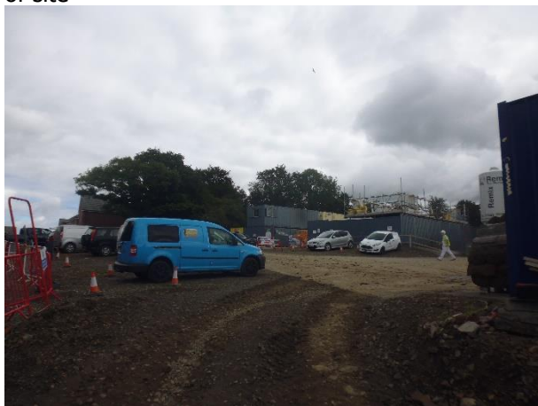
Photo 1: Construction compound in northern half of site
