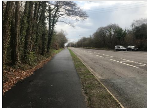
A48 – Looking East
