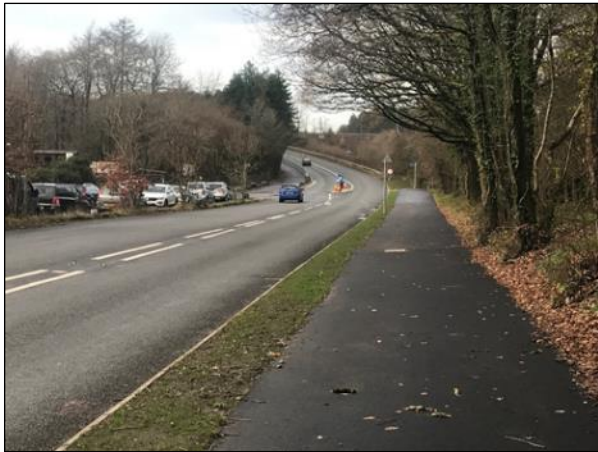
A48 – Looking West
