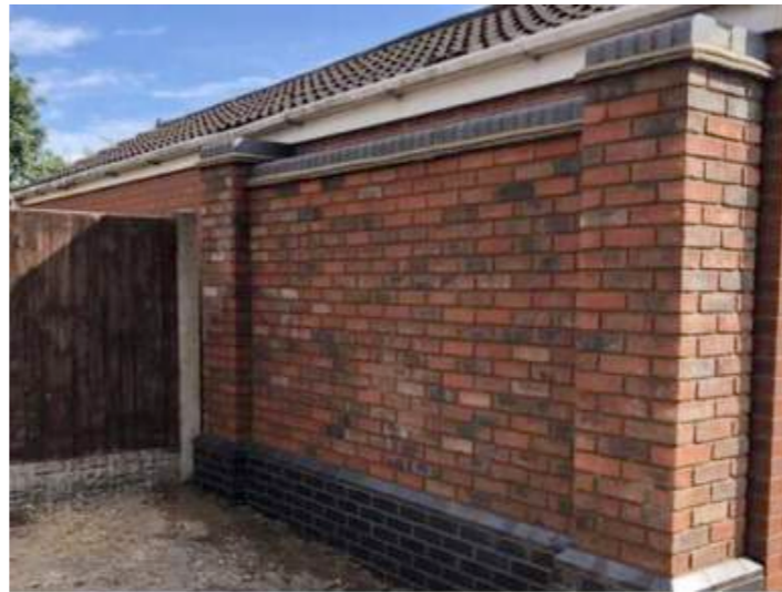
1.8m brick walls with detailing in staffordshire blue for rear garden boundaries facing the public realm.
