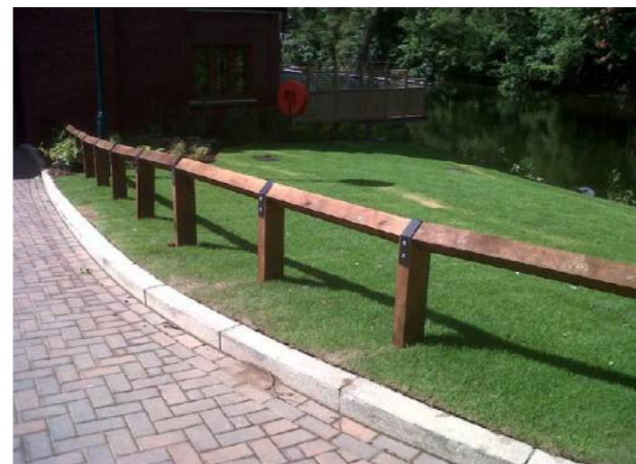
Timber knee rail fence is proposed as separation between private and public spaces towards the public open space.
