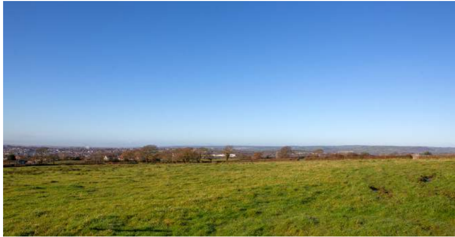
Viewpoint 5 - The 3M water tower is a key landmark visible from the site to the south-west, with views of Gorseinon to the south-west and west. Existing residential properties run along the south edge, with vegetative screening varying from minimal to fairly dense.
