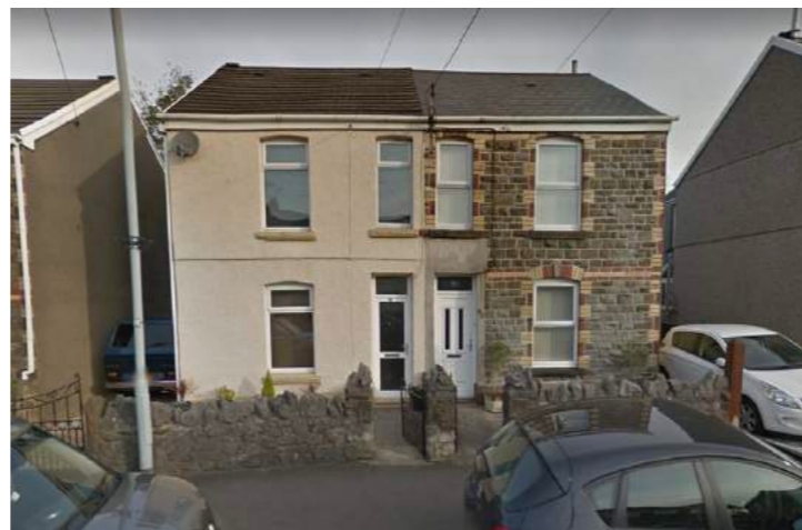
1 - Historic development along the A4240 with small detached and semi-detached properties in stone and render.
