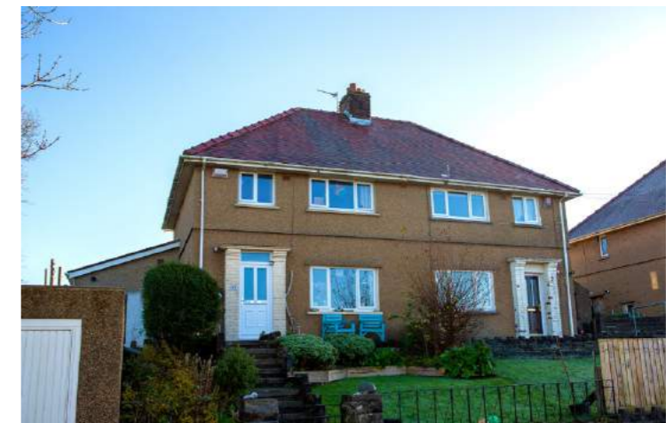
2 - 1930s development with typical semi-detached large properties featuring hipped roofs and chimneys in a mixture of pebble dash, brick and white/off-white render; generous front gardens often used for parking to the front of the property
